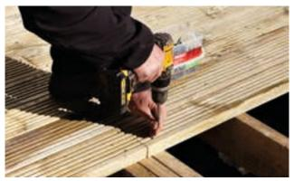
Pre-drilling pilot holes for fixings (nails or screws) prevents splitting at board ends. When installing hardwood, pre-drill all fixing points.
