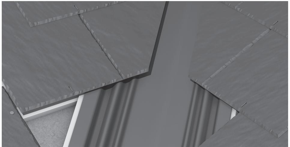
Fig. 1 – Raking cut slates laid with GRP valley trough
