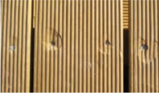
Damage caused by misuse of a high pressure nail gun
